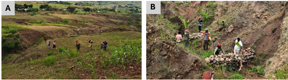
Figure 40: AMU-IUC demonstration workshop on gully check dam construction, Layo Terga Case 1, August 2025. (A) Farmers collaboratively transporting stones to the gully, (B) check dam construction under expert guidance. Photos by author, [August 2025].
