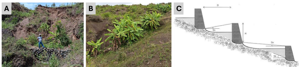
Figure 3: Examples of gully interventions in Shafe catchment: (A) Loose rock check dam constructed transverse to the gully channel. (B) Example of a vegetative intervention: Banana plants established on the gully floor. Photos by author, [A: August 2025; B: September 2025] and (C) A schematic longitudinal section of check dam dimensions, including height ( H ), horizontal distance between dams ( D ), gully bottom slope ( S_b ), and slope gradient connecting spillway and upstream dam foot ( S_n ), simultaneously illustrating the stepped topography. Figure taken from Nyssen et al. (2004)
