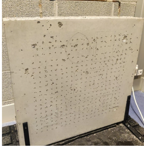
Figure 28: Surface damage observed after repeated projectile excitation with steel spheres. Although the LDV measurement itself is non-contact, the current excitation mechanism produced local impact marks and small surface indentations on the concrete specimen. This illustrates that the present configuration should be regarded as a non-contact vibration measurement setup with mechanical impact excitation, rather than as a fully non-destructive inspection method.
