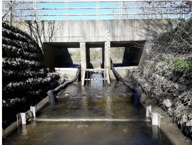
Figure 8 Return crab trap on the Melsenbeek (Provincie Oost-Vlaanderen, 2021)
