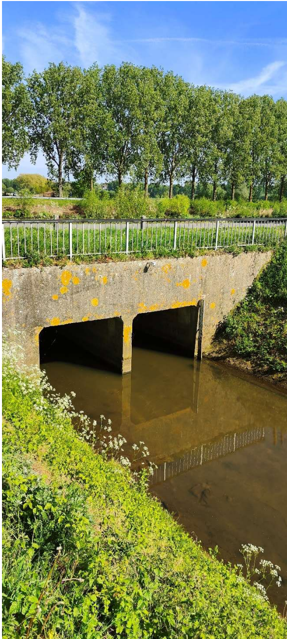
Figure 18 Perspective of the steep embankments
