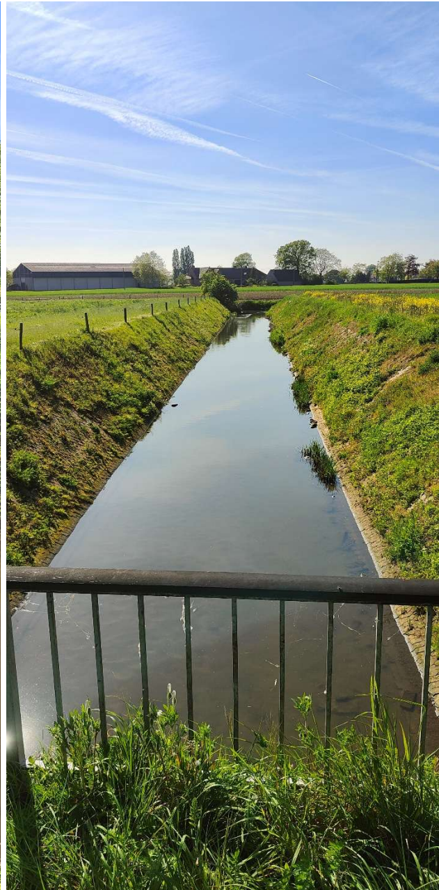
Figure 19 View of the location from the bridge structure
