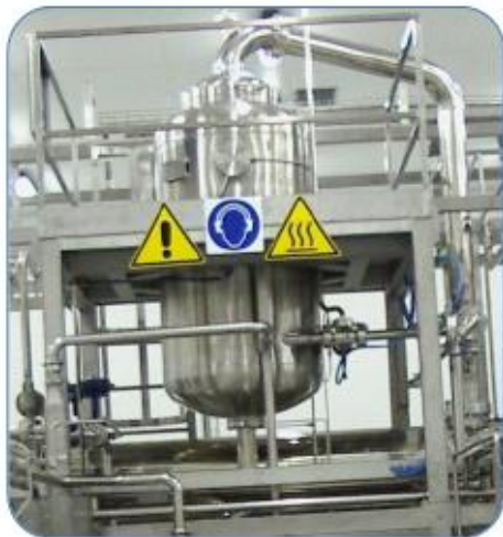
Figure 3-8: Deaerator used in Reggiani (manual)
